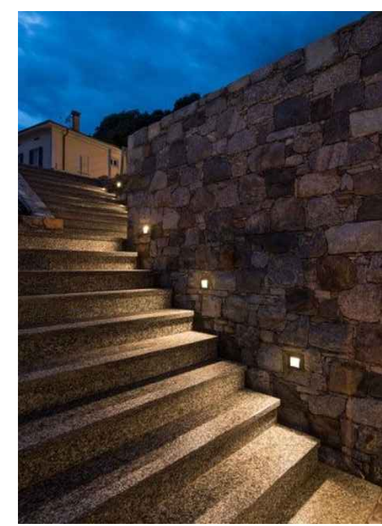
Building mounted light
